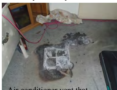
Air conditioner vent that dropped out of the ceiling
